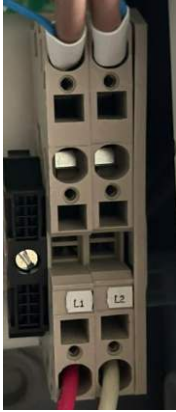
Figure 4.10 AC Connection Area of Inverter
